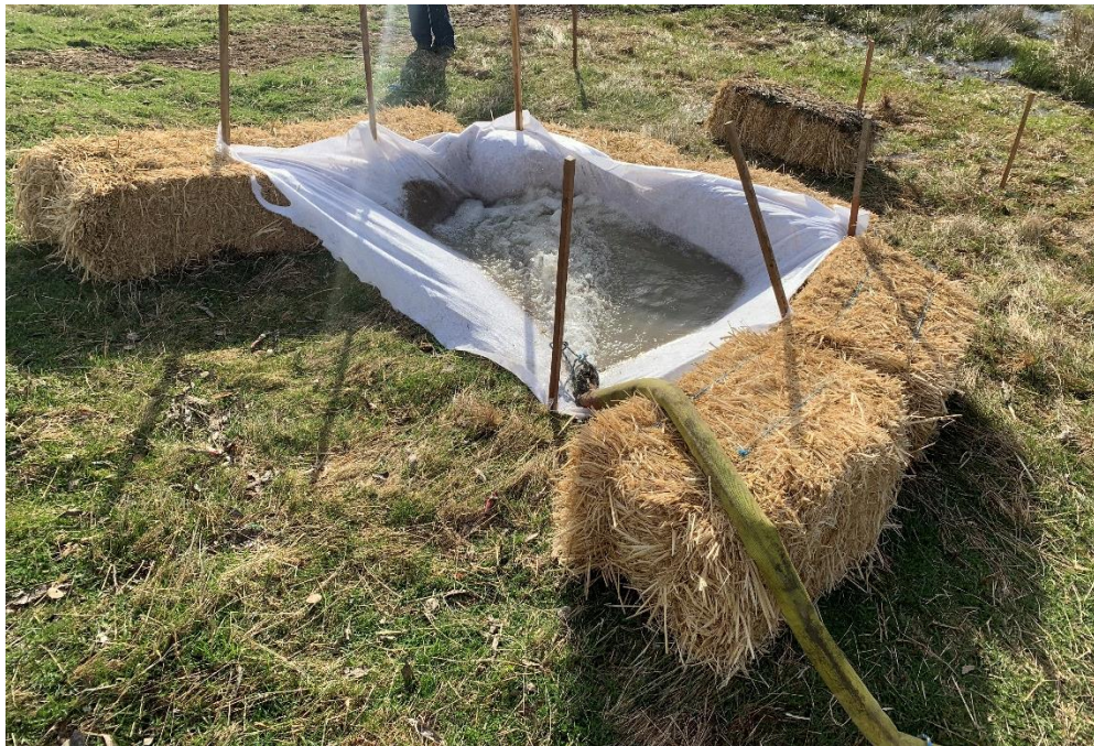
Figure 5: Standard Installation of Geofabric Filter Dam
