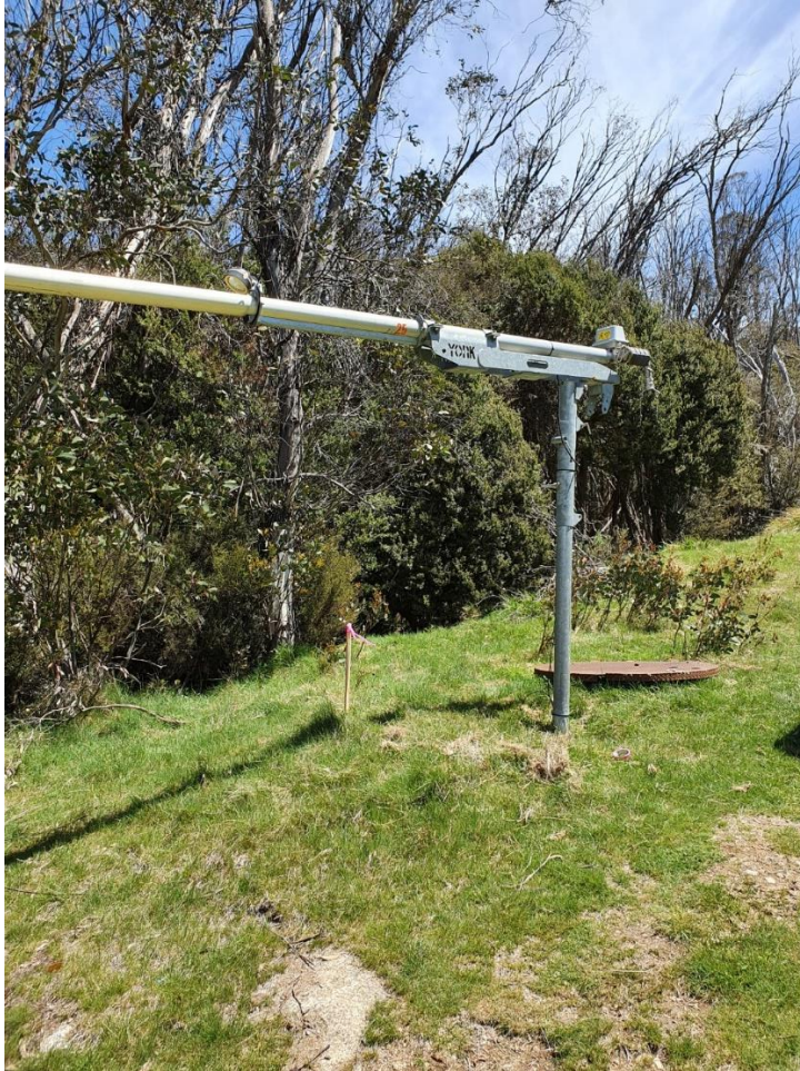
Photo A4: TT10 #2 (Easy Does It skiers right) – replacement of existing lance gun with TT10 fan gun
